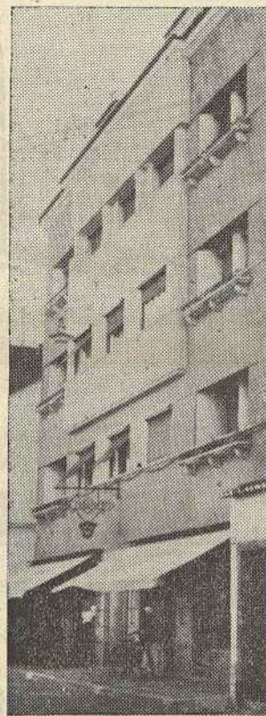
Fachada principal do Terrabela-Hotel
